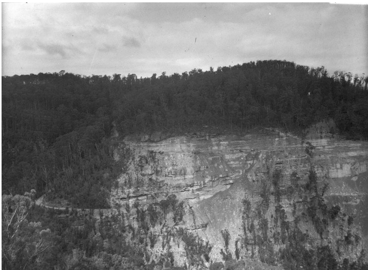
State Archives of NSW image - NRS-4481-3- [7/16112]-St30079. Government Printing Office 1 – 43417. Mt Tomah section of Main Road no 184 [From NSW Government Printer series: Main Roads] Between 01-01-1947 to 31-12-1947.
